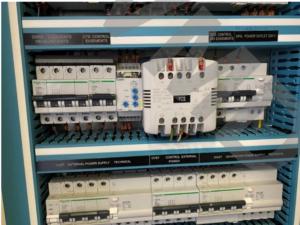
Power Control Unit UPS & Power Generator (door open)
